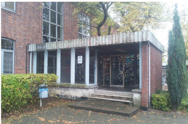
Figure 12. Entrance 1 at the northern side of the test building.
