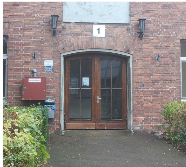
Figure 13. Entrance 2 at the southern side of the test building.
